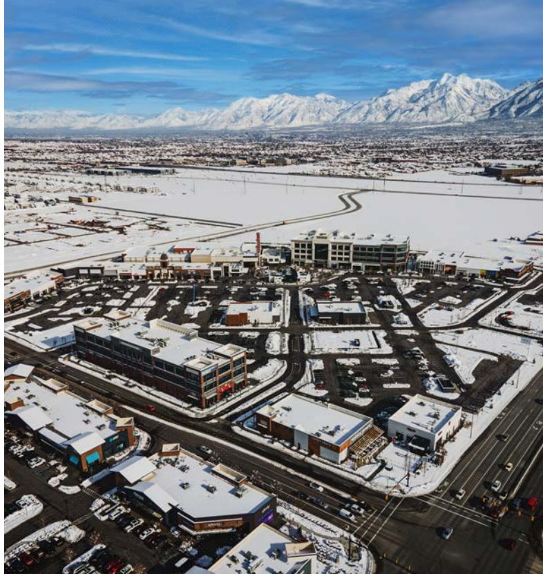
13400 S Mountain View Corridor
