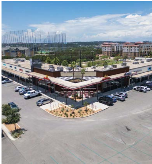
Shops at South Rim 38,825 SF RETAIL | TEXAS
