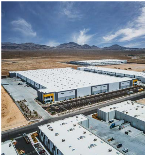
Northgate Distribution Center 180 ACRES INDUSTRIAL | NEVADA
